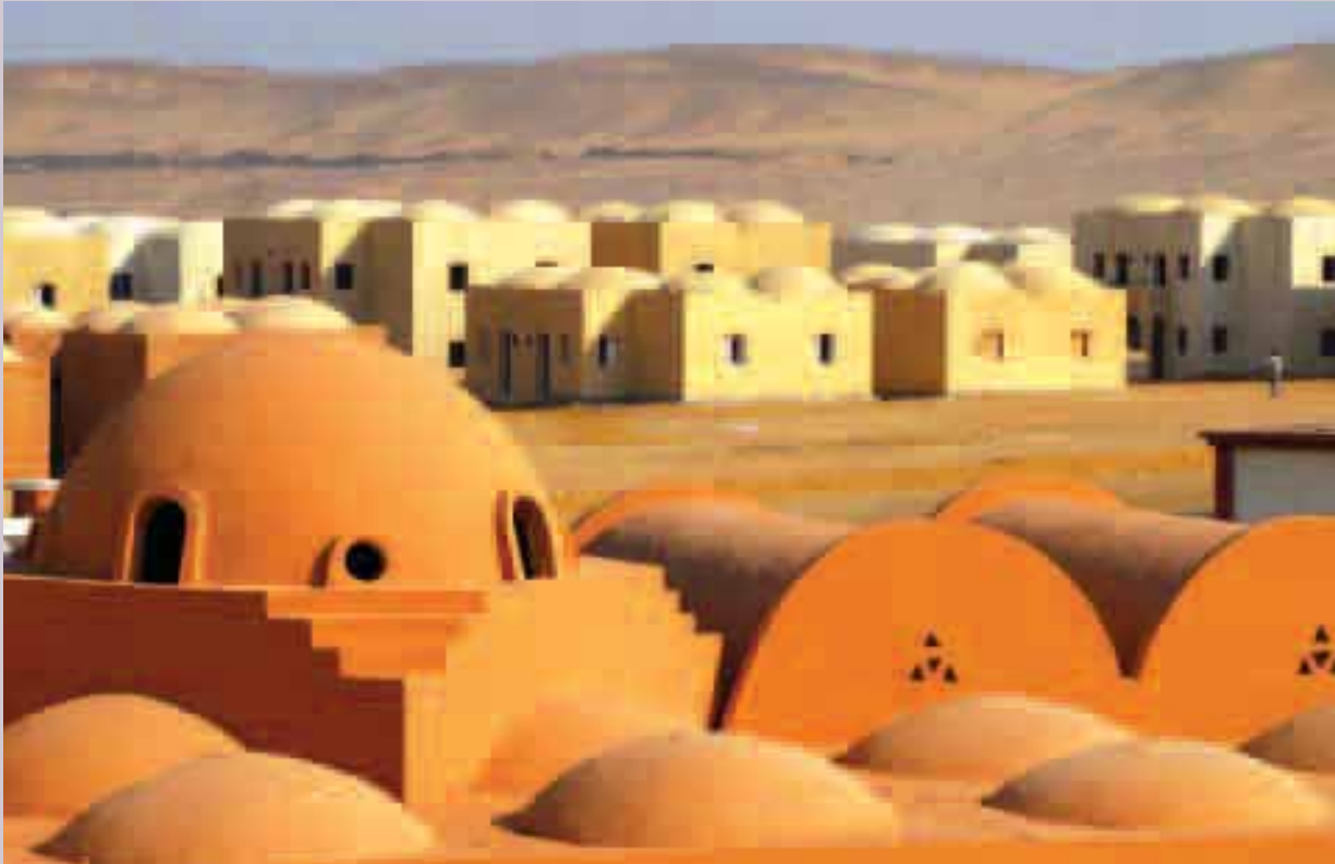
▲ Orascom affordable housing in Haram City, Egypt. Photo courtesy of Orascom
