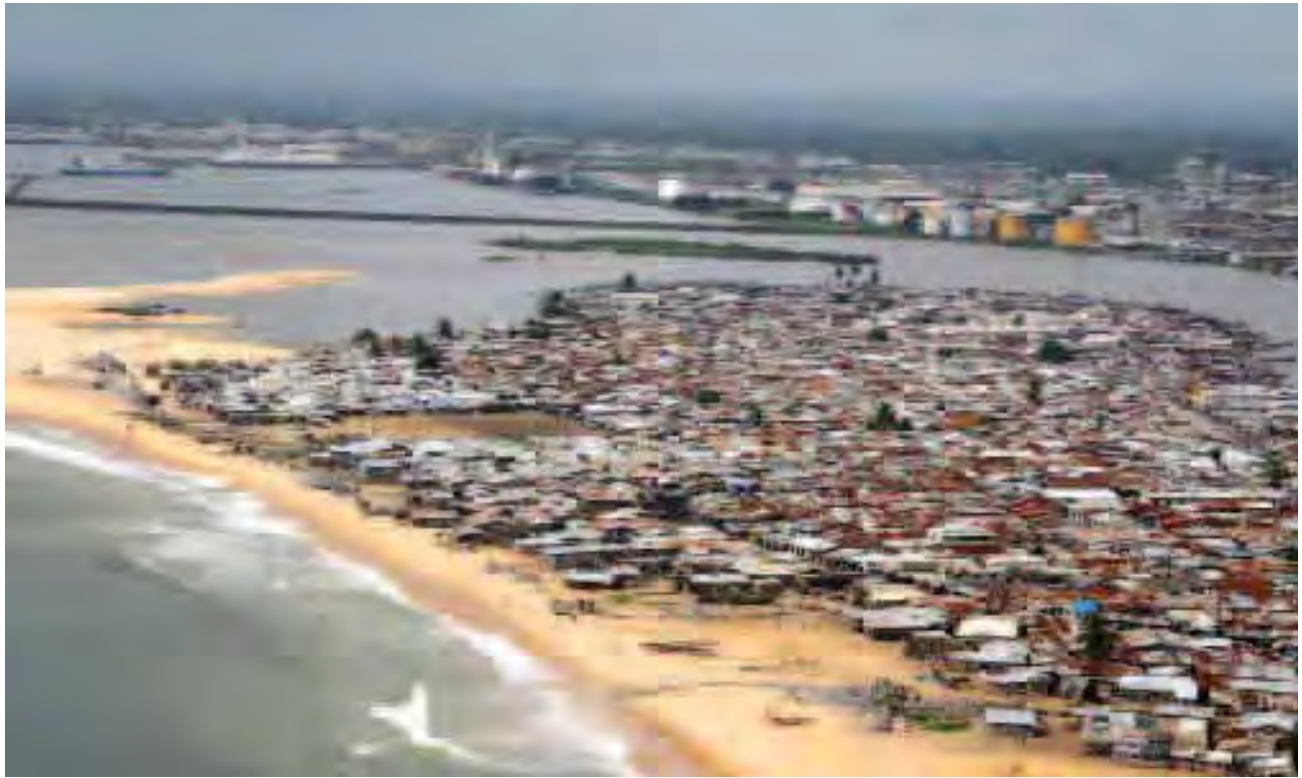
▲ West Point slum, Monrovia, Liberia. An example of an informal settlement vulnerable to surge flooding. ©Tugela Ridley/IRIN
