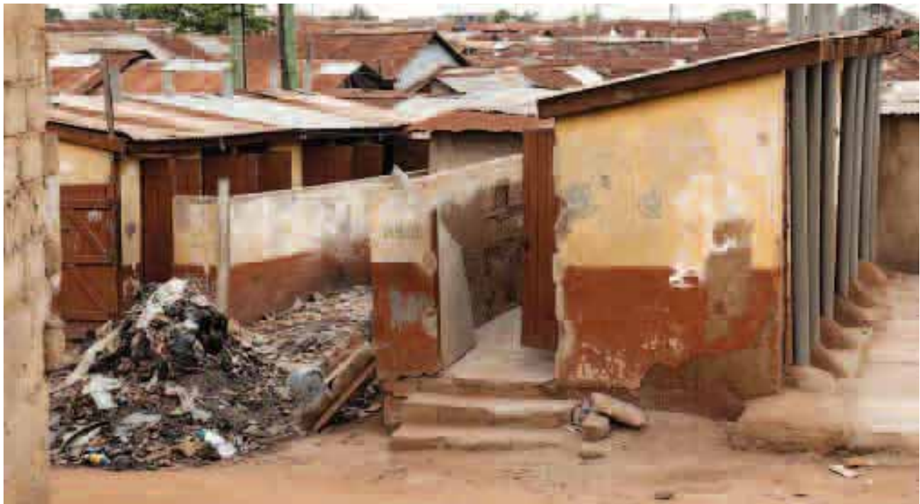
▲ Accra, Ghana. Communal toilet blocks in an informal settlement. ©Gordon Dixon/iStockphoto
