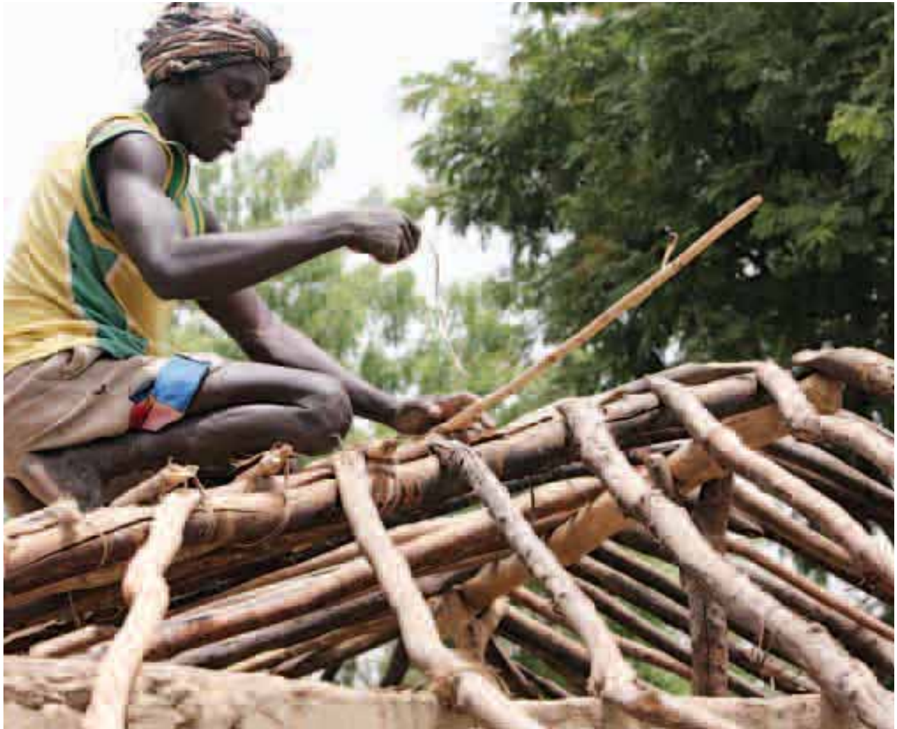
▲ Roof construction, Central African Republic. ©Anthony Morland/IRIN
